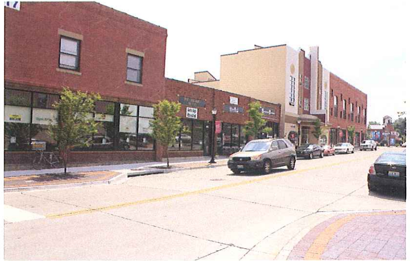
Along-range strategic planning has resulted in many achievements in downtown Lee's Summit. Among them is the new streetscape. This view is along southeast Douglas Street.
